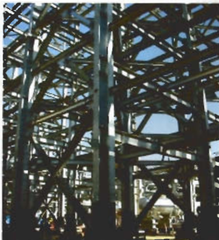
A Khurais project for which the company was contracted
